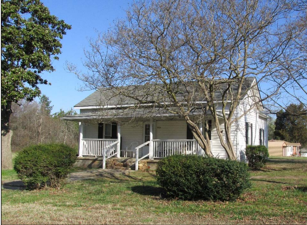
Figure 9. Rich Hatchett House, front and east elevations.
