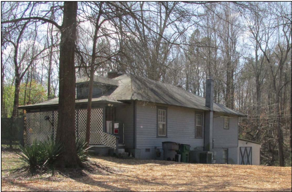
Figure 12. Pressley Farmhouse, front and north elevations.
