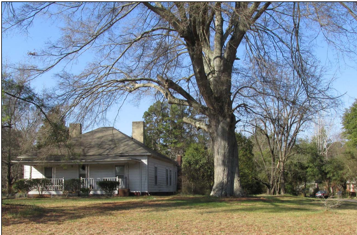
Figure 5. Pink Graham House, front and north elevations.
