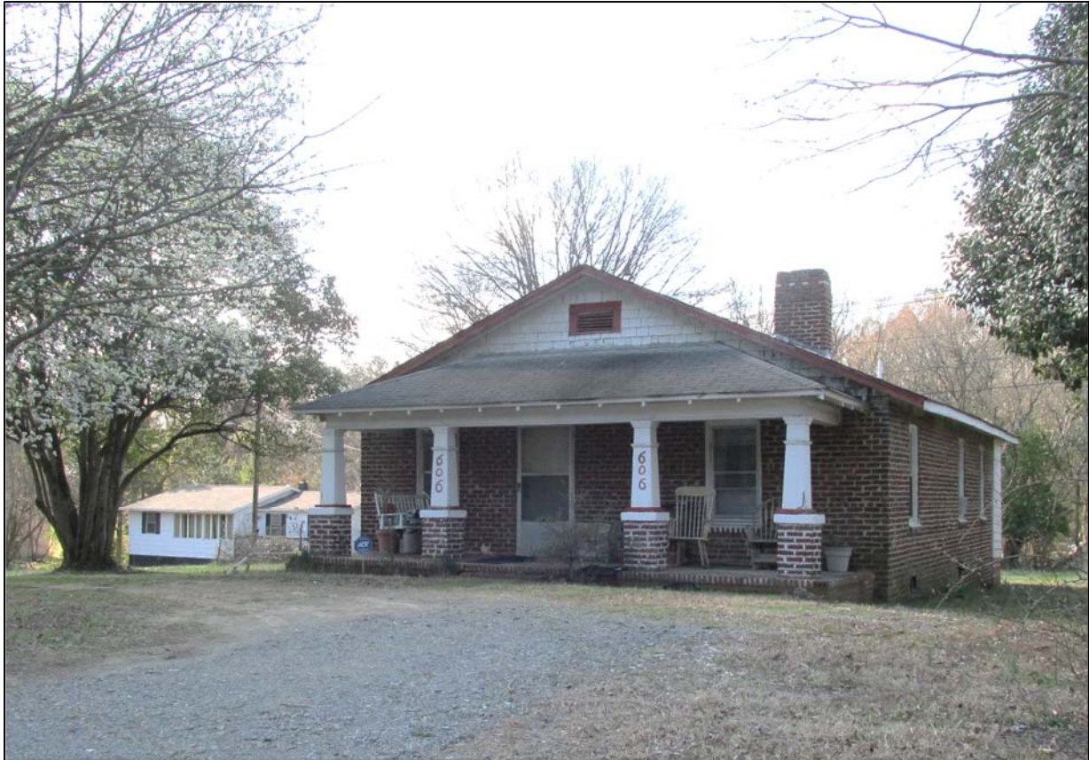
Figure 13. Rowland-Clay House, front and north elevations.
